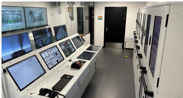
Figure 7. The K-Sim Engine MAN B&W 5L90MC VLCC L11-V engine room simulator setup at the Copenhagen School of Marine Engineering and Technology Management (Teknika).
