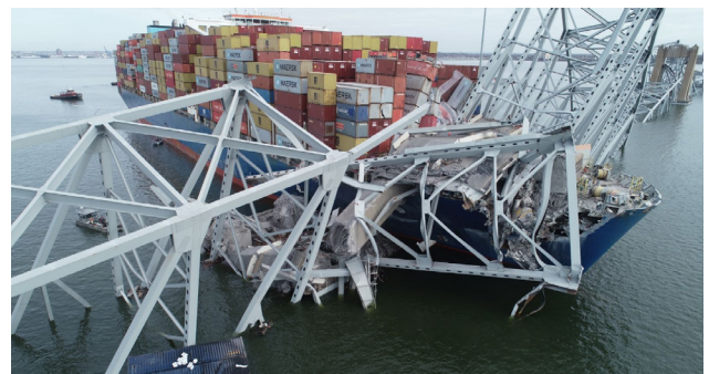
Figure 2. MS Dali collision with the Francis Scott Key Bridge [7, p. 232]. The main engine shut down automatically due to low cooling-water pressure. As the main engine was no longer rotating the propeller, no wash was provided across the rudder. This meant that the crew could not effectively steer the vessel [7, p. 153].
