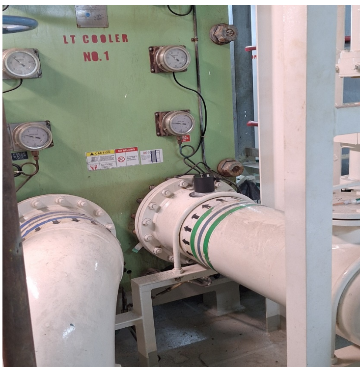
Figure 2.2 Ultrasonic transducer installed on top of pipe leading to low-temperature (LT) cooler No. 1.
